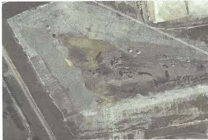
Sandy Pines Site (5/16/13) TMS# 085-00-00-065 Site visited 5-8-13. Residential yard debris currently staged at this site
