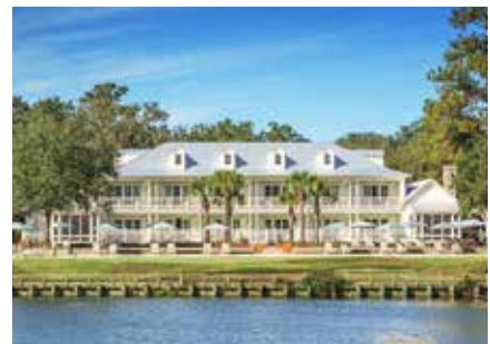
Windows and doors should be organized systematically to create consistent building bays
