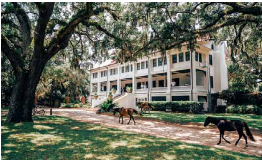
Large front porch and additional living spaces added across the front of the building
