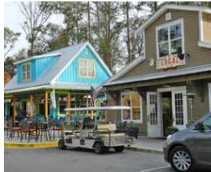
Small-scale commercial building precedent
